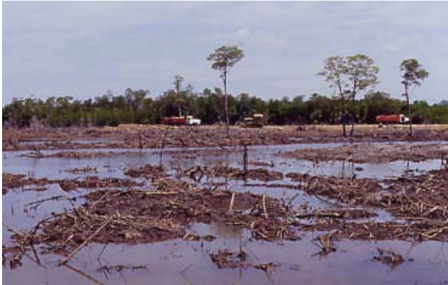
Hotel construction, Fiji
