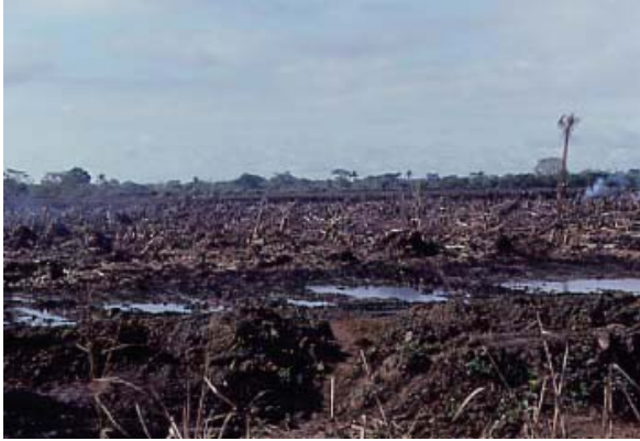
Shrimp pond construction, Ecuador
